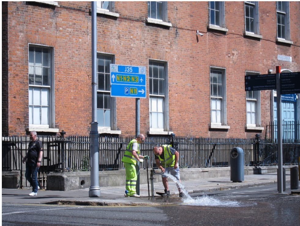
Figure 5.9.4: Watermain Flow and Pressure Tests June 2018
